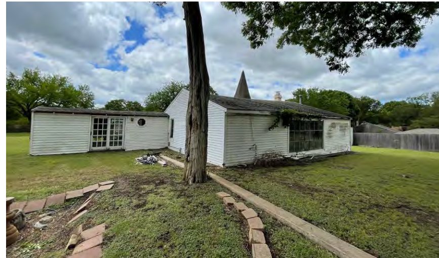
View of addition and hallway, view facing southwest
