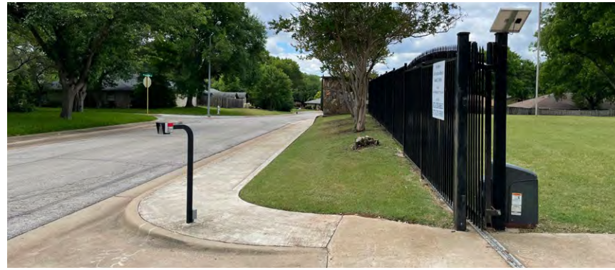
View facing south showing entrance gate
