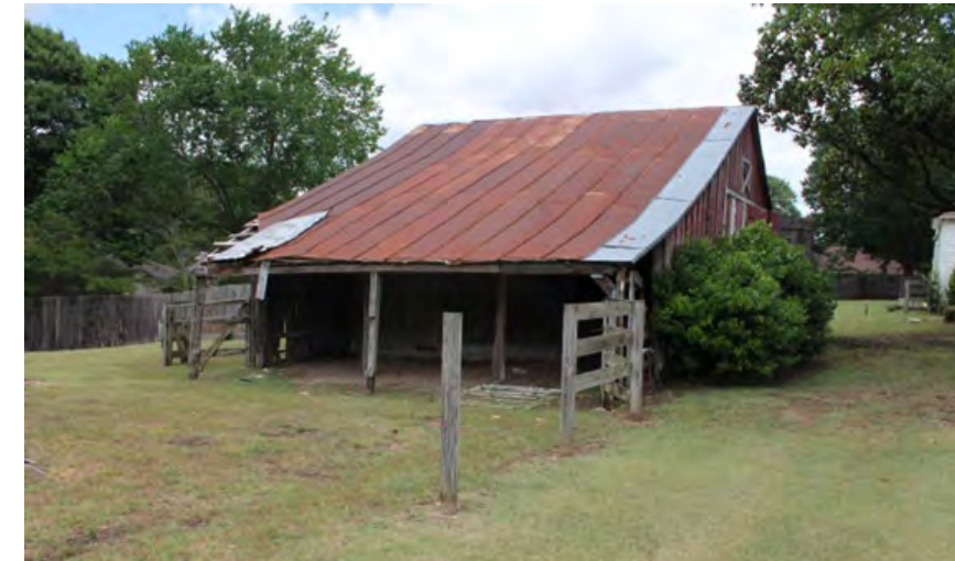
South elevation of barn, view facing northwest
