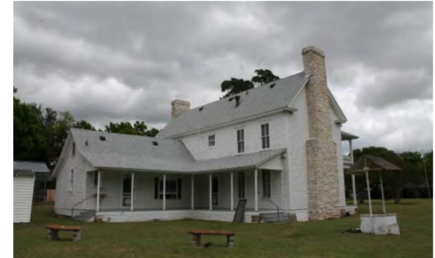
South and West elevations of farmhouse, view facing northeast
