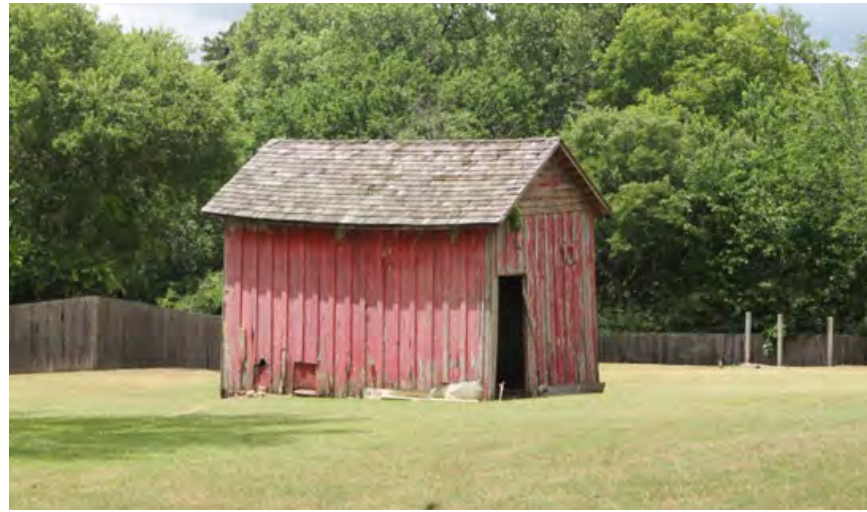
East facade of Curing Shed, view facing southwest
