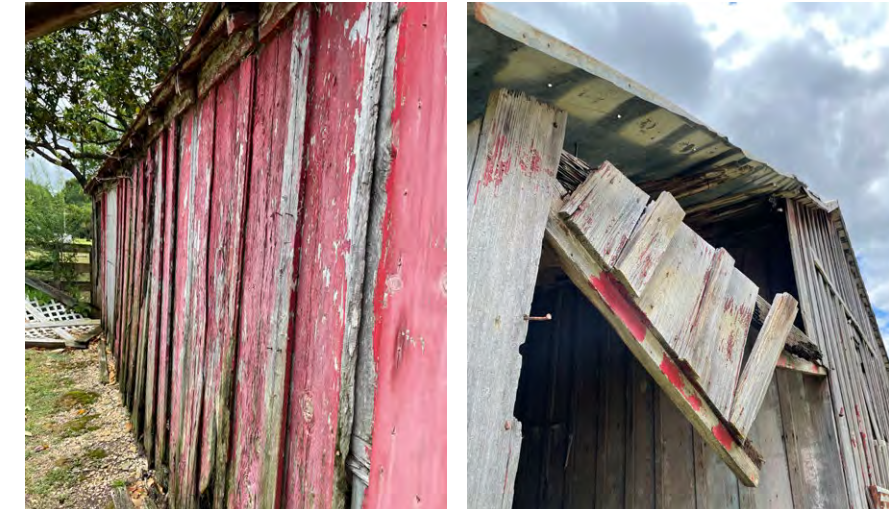
Milking Barn North Facade
