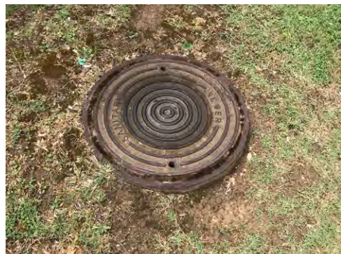
Sanitary sewer manhole on southwest corner of property
