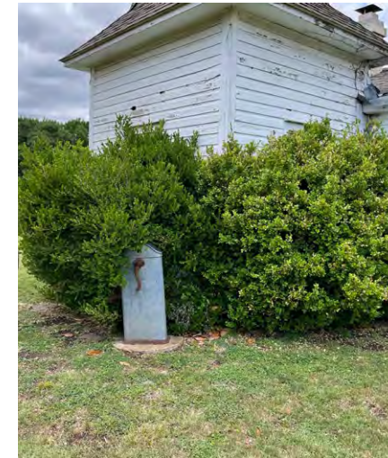
Water Tower exterior, view facing southwest
