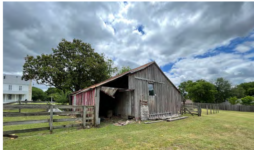
West elevation of Barn, view facing southeast
