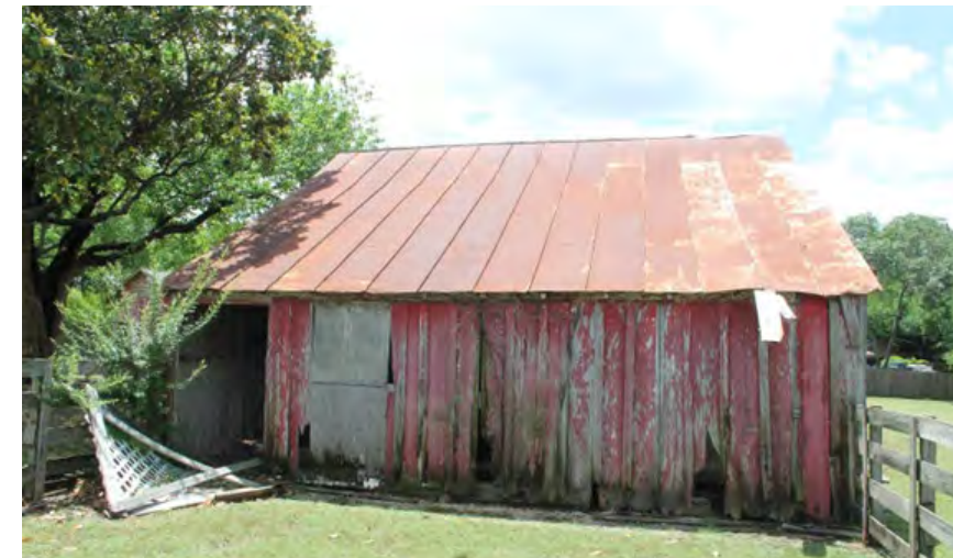
North elevation of barn, view facing south
