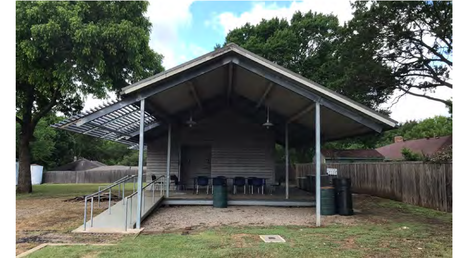
View of restroom structure, view facing west
