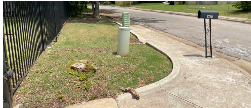
View of renovated sidewalk, view facing north
