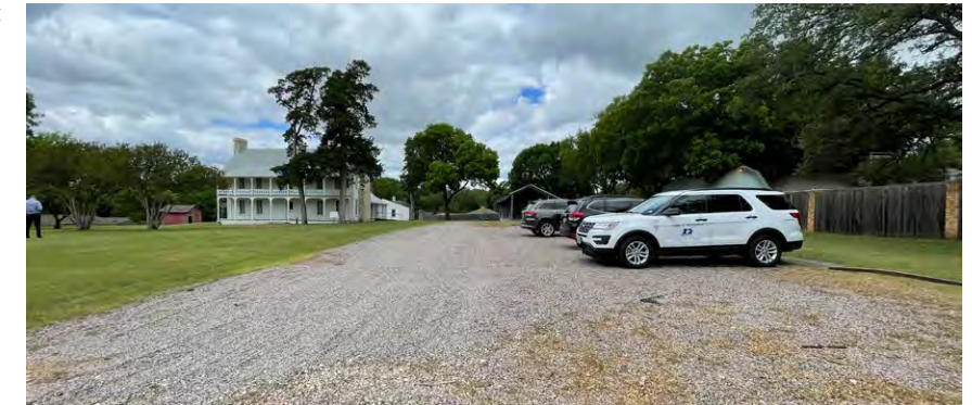
View facing west of parking lot
