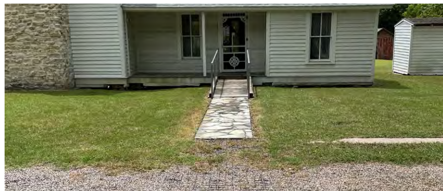
Main House north facade, showing ADA ramp and side entrance, view facing south
