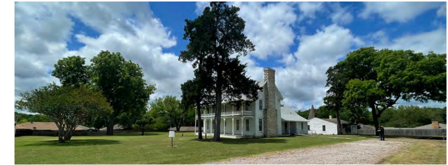
1 View from parking lot toward Main House, facing southwest
