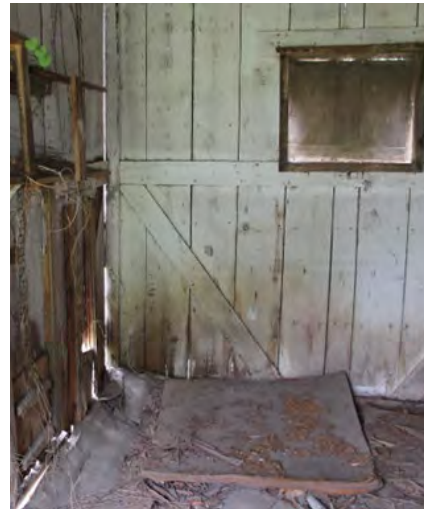
Curing Shed interior view
