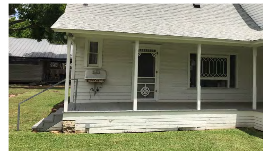
Back Porch East Stairs Detail
