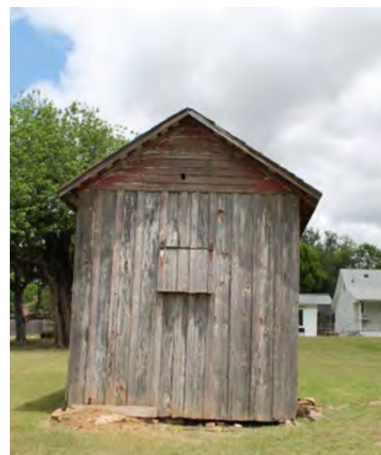
South facade, view facing north
