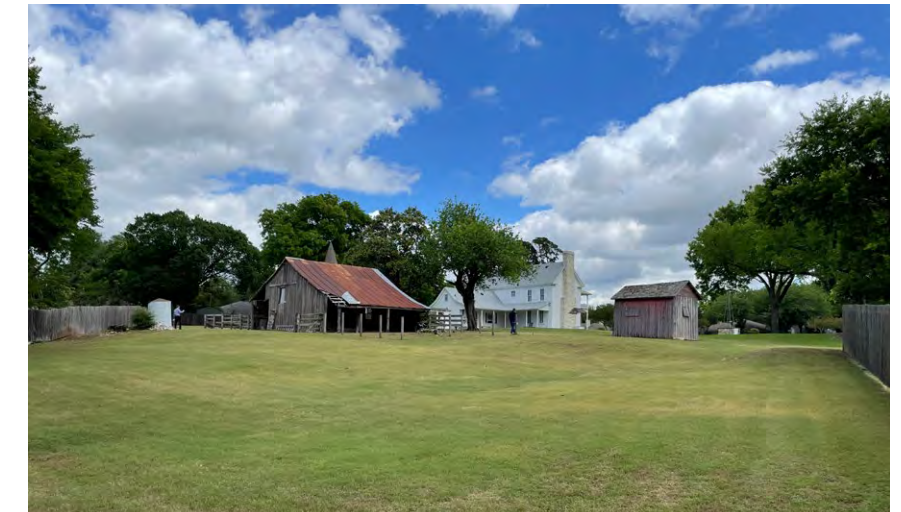
4 View from back lawn facing northeast, showing back facades of Milking Barn and Curing Shed
